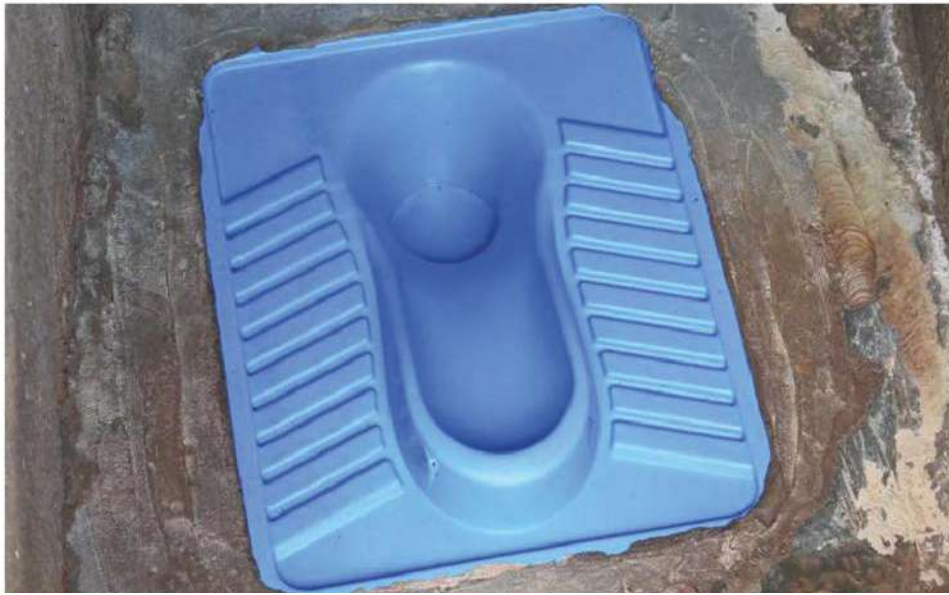
A SATO toilet bowl in Bar Agulu village, Siaya County. [Denish Ochieng, Standard]
